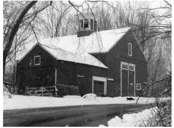
Photographer Richard Auger of Whitinsville: the former Armsby Barn
